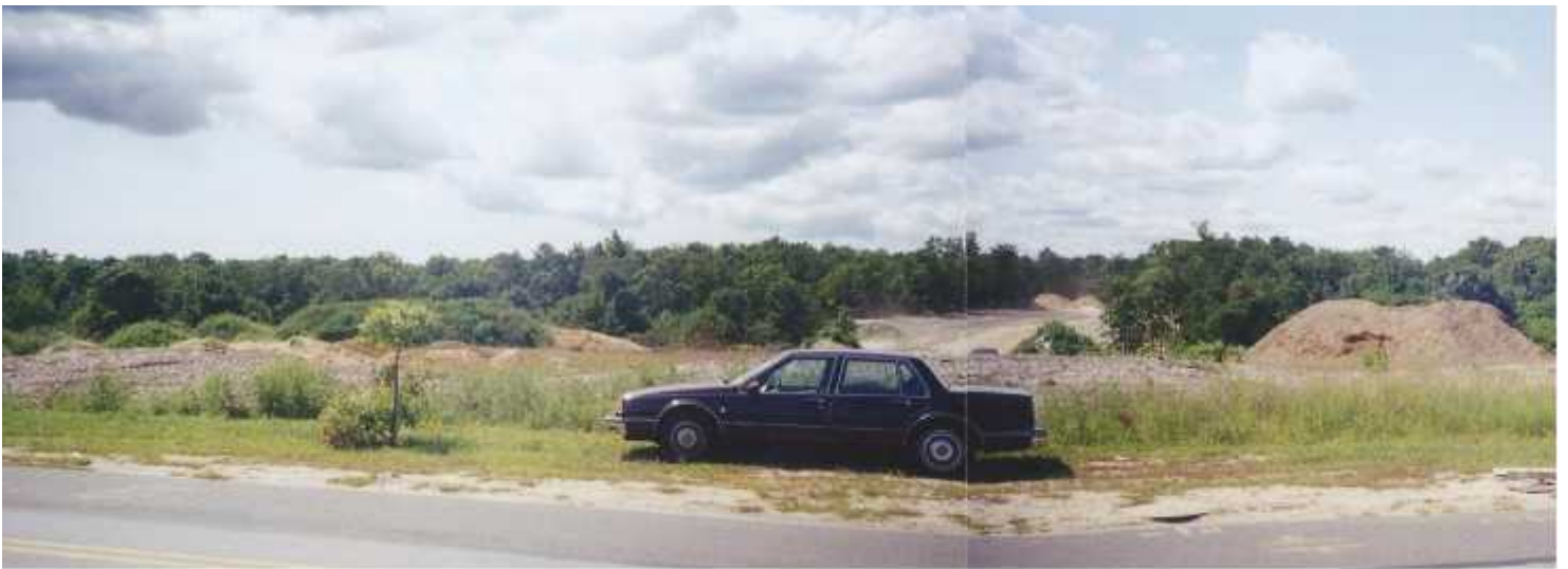
AND THE WORK BEGINS.....
